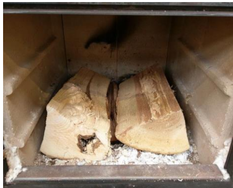
Figure 12 Logs Laid in Firebox
