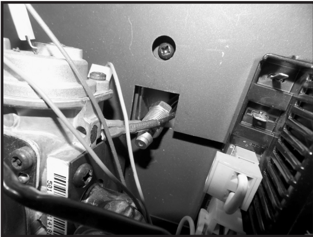
Figure 69: Square slot for insertion and removal of pilot assy.
