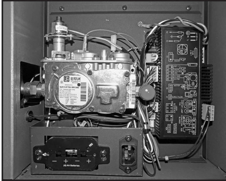
Figure 44: Valve & IFC module location.
